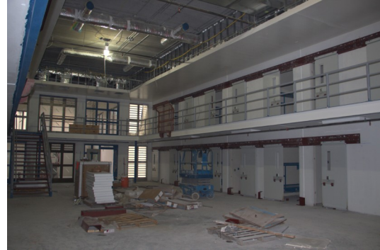
Left: Aerial view of the new jail towers which will nearly double the CCSO inmate capacity to 2,360. Above: Cell doors have just been installed in one of the new housing units. The new housing units will likely be completed in early 2013. Photos by: Chief Deputy Roy Harris and Michelle Gavin
