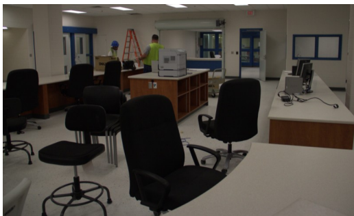
Above: The CCSO's telecommunications staff and engineers are putting the final touches on the new pre-booking area. It should be complete later this fall.
